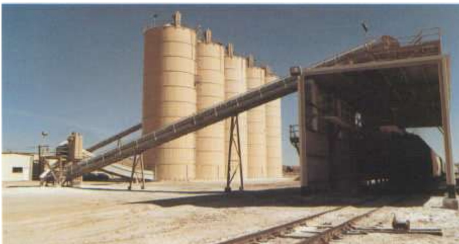
A 100 ton railcar can be loaded with soda ash every 15 minutes in this automated terminal.
